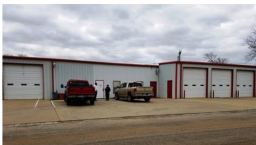
Figure 121: Bullard VFD, Station 2
